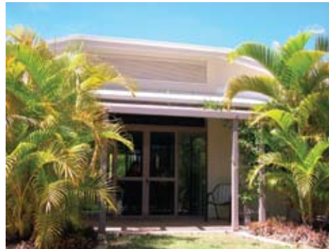
Patio at the dining room (W) with through-view to the verandah (E). Note the ventilation louvres above, to the attic space.
