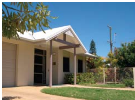
Entrance, facing N/W, well shaded.
