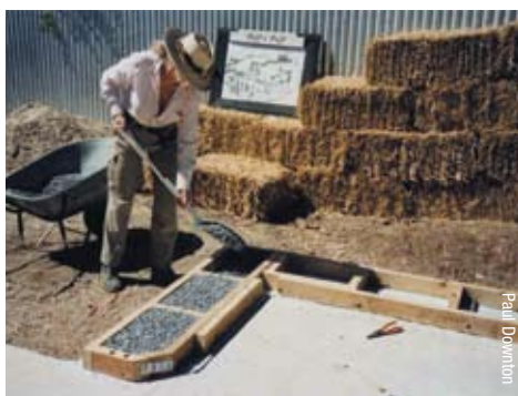
Ladder frame being filled with pea gravel prior to frame and bale placement.
