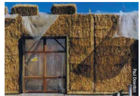
Window set towards outside face of wall.
