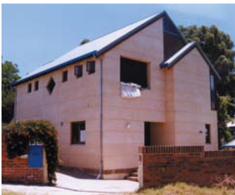
Perth rammed earth home.
