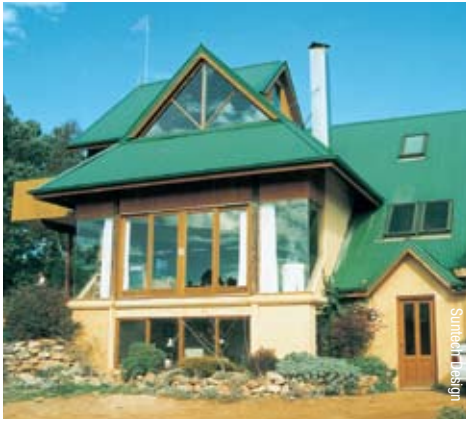
High mass lower level (earth bermed pre-cast concrete) and low mass upper levels (insulated timber framed or AAC block) are combined to optimise use of embodied and operational energy.
