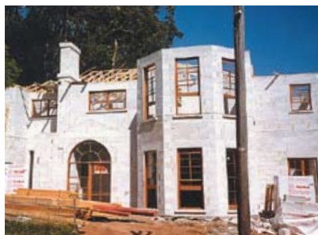
Block construction showing two storey house.
