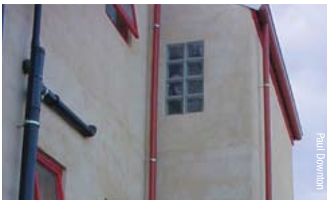
External plumbing was chosen to reduce loss of internal space and avoid potential problems with wall cavities, and adopt the use of HDPE plastic in the construction.
