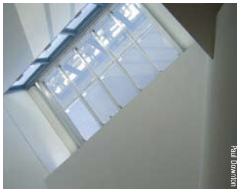
Skylit central stair and liftwell uses integrated semi-transparent PVs as roofing material.
