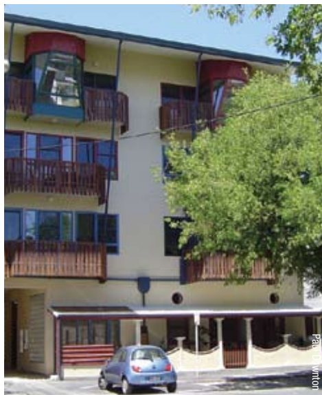
An apartment building where the eaves shade the whole north façade during the middle part of the day.
