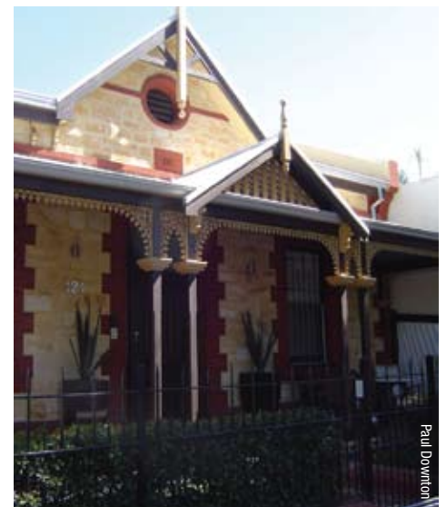
Colonial cottage with vents to main roof and gabled verandah.
