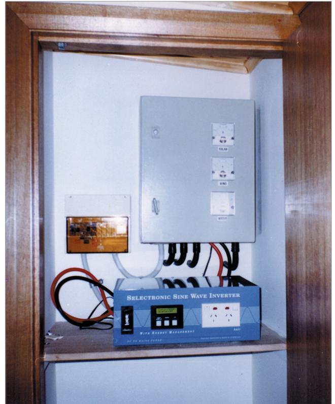
Install inverters where there is suitable ventilation, no direct sunlight and easy access.
