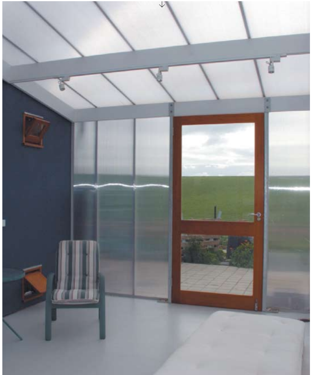
The glasshouse is the home's only source of heat.
